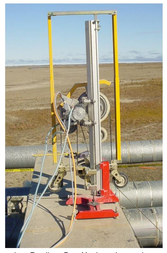
Pictured on Prudhoe Bay Alaska, wire sawing on the Alaskan Pipeline.
